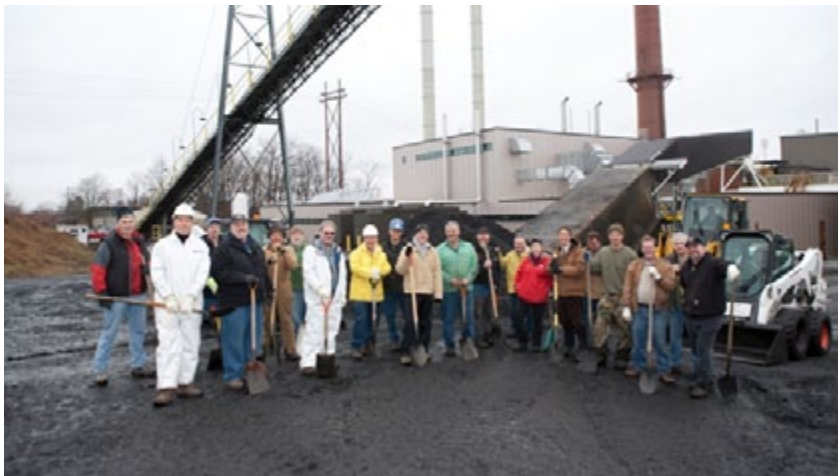
Cornell employees shovel the last loads of coal into the Central Energy Plant.
