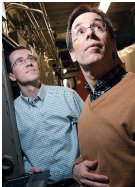
Mark Howe, Program Manager for the Energy Conservation Initiative, left, and Lanny Joyce, Director of Energy Management in Cornell's Department of Energy & Sustainability, right, examine the Cornell Store's recently updated HVAC system.
