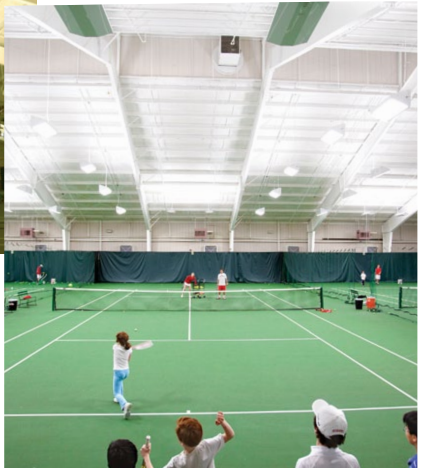
Cornell's Reis Tennis Center before and after lighting retrofit. The new lights are twice as bright and far more efficient, using 70 percent less energy annually compared with the old metal halide lights. They will also save $20,000 per year on energy costs.
